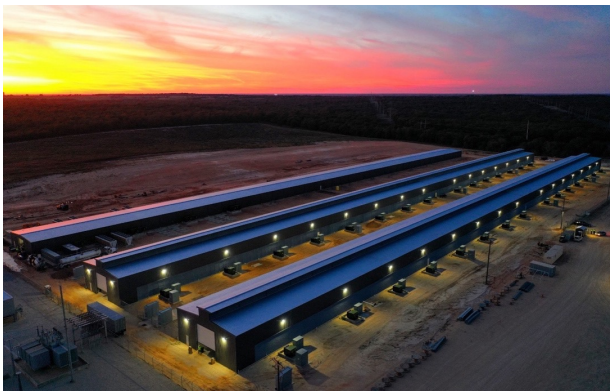
Whinstone facility, Rockdale | Riot Blockchain imagery reproduced in Castle Island Ventures, Texas Blockchain Summit, October 2021, p. 5 [P5]. Historical facility context.
